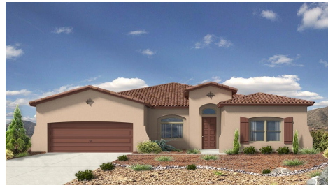
Victoria Mission Tile Roof
