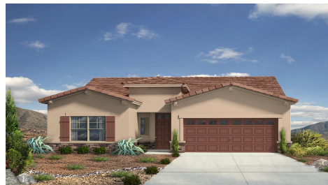
Selena Craftsman Shingle Roof
