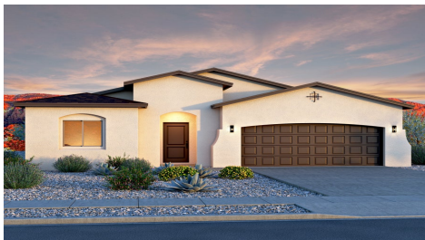
Tabitha II Mission 4th Bedroom Shingle Roof
