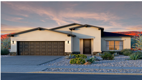
Tabitha II Craftsman Shingle Roof
