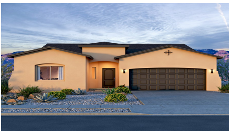
Selena Mission Shingle Roof
