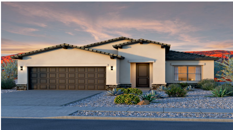
Tabitha II Craftsman w/Stone Homes may be built in reverse of plans shown, depending on site conditions. Minor architectural changes may be made occasionally at the option of the builder. Printed material is not date stamped. Prices are subject to change. Please reference Abrazo Homes' website for most updated and accurate pricing and information. Please contact your Sales Consultant for details.
