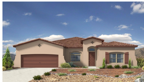
Victoria Mission Tile Roof
