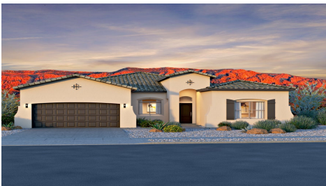
Victoria Mission Tile Roof
