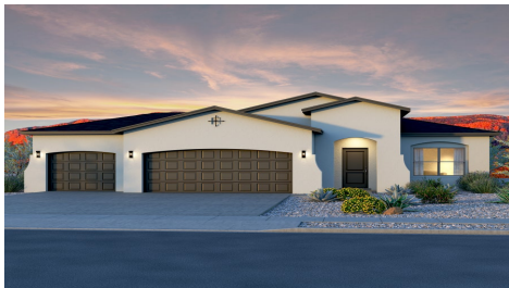
Tabitha II Mission 3 Car Shingle Roof
