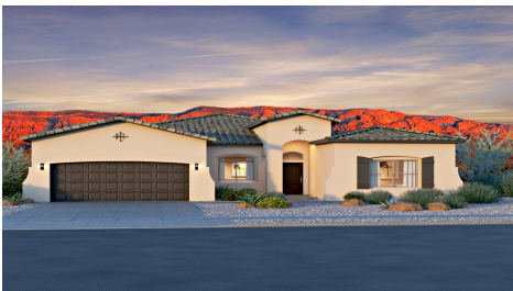
Victoria Mission Tile Roof
